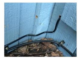
6.6 EZ-Bend cable fastened to an existing conduit using cable ties.
