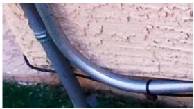
6.7 Installing EZ-Bend cable through a conduit into the attic of a home.
