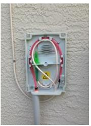
6.10 EZ Bend Cable terminated on the interior wall of the living unit.
