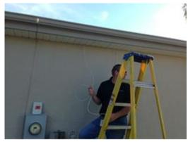
6.9 EZ Bend Cable can be fastened to masonry walls using shark tooth anchor clips<sup>3</sup> or similar fasteners.
