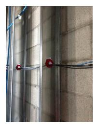
6.3 EZ-Bend cable can also be stapled or fastened with cable ties as shown in the following photos. As mentioned before, only *ruggedized* versions of EZ-Bend cable can be stapled. Standard CAT-5 cable staplers (Arrow T25, Acme 25A, or equivalent) and rounded cable staples (Arrow T25, Acme 25A, or equivalent) must be used to staple the cable. EZ-Bend cable can be routed (but not pulled) around corners and moldings without the use of bend limiters.
